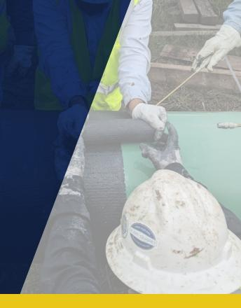
This sacrificial outer laminate system protects pre-approved anti-corrosion field joint coatings and mainline coatings such as FBE, liquid epoxies, shrink sleeves, and tapes. ScarGuard® minimizes the need for costly repairs after pull back and provides robust protection of the underlying pipeline coating.
